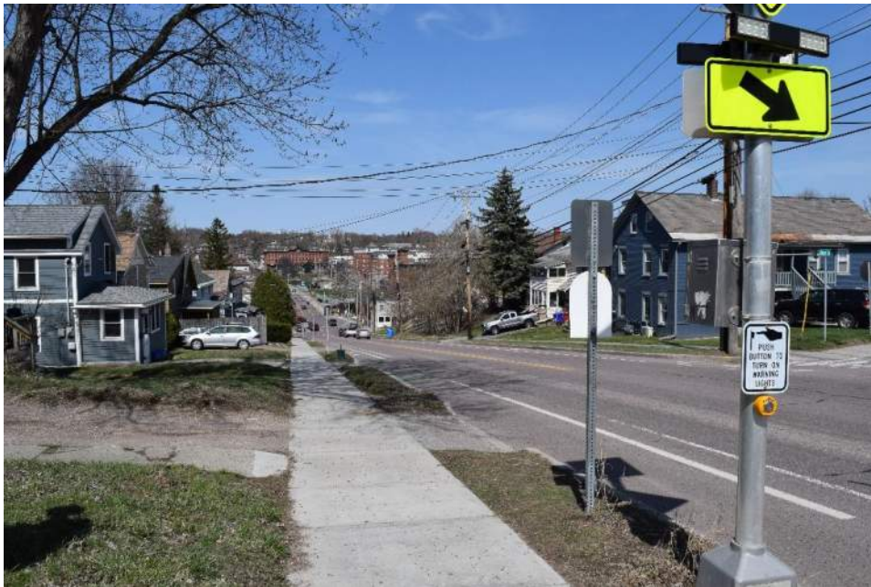
Photo 82: View towards the bridge from the intersection of Colchester Avenue and Chase Street.
