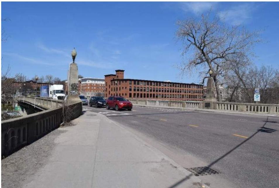
Photo 12: Bridge approach from Burlington. Map ID 9.
