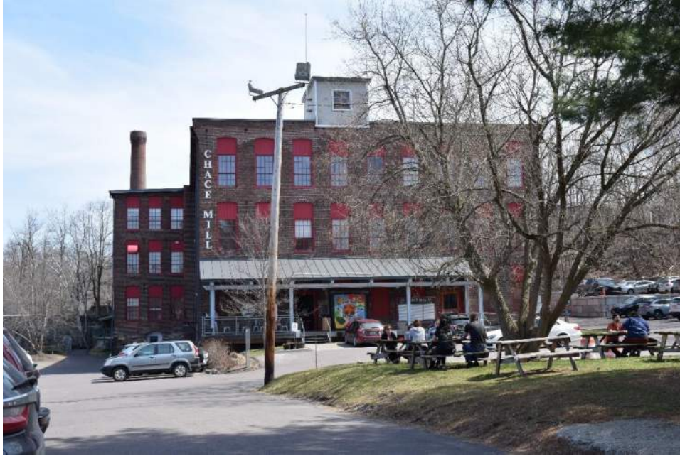
Photo 118: 1 Mill Street façade. Map ID 99.
