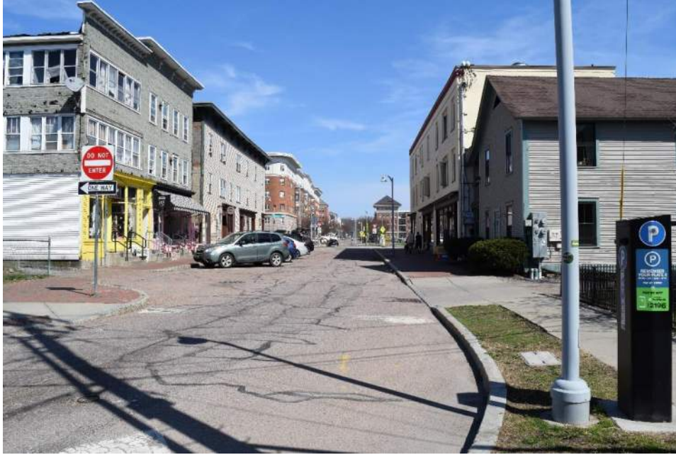
Photo 136: Streetscape facing towards Main Street.
