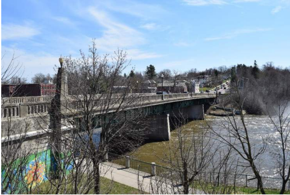
Photo 15: Bridge showing the decking and piers. Map ID 9.
