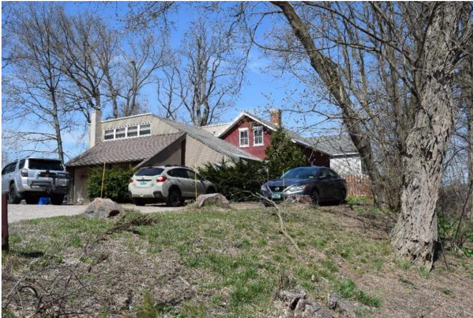
Photo 48: 1970s addition to 352 Colchester Avenue. Map ID 37.
