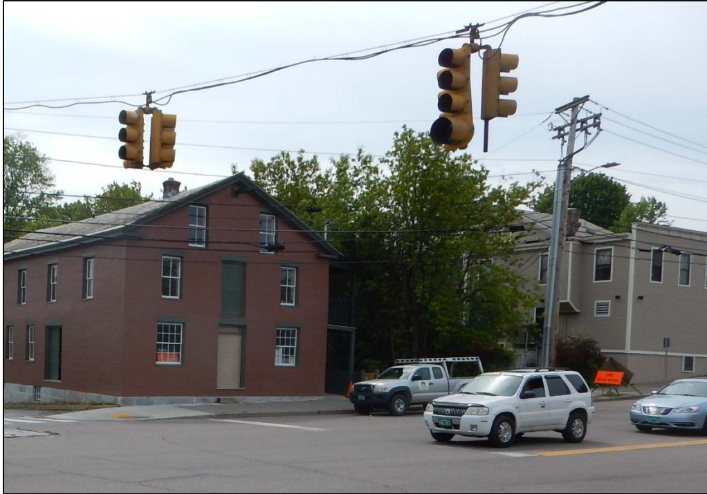
Photo 5. Overgrown area between Structures 20 and 21 that once contained a carriage house from 1894 to 1906, a shed from 1912 to 1919 and a garage in 1926, as depicted on the Sanborn maps. View to the east.
