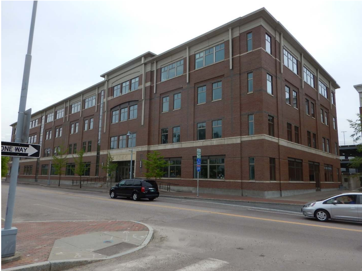
Figure 37. View looking southeast at 10 East Allen Street, 2017.
