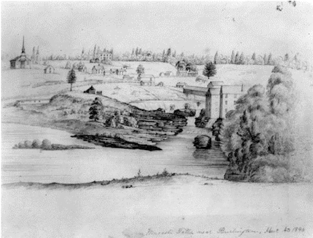
Figure 2. Winooski Falls near Burlington, Drawing, 1840. Project area, including the covered bridge over the Winooski River, is seen at right center in this view ( www.uvm.edu ).
