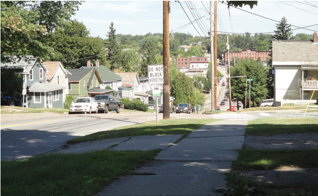
Figure 9. A similar view, looking north, 2016.
