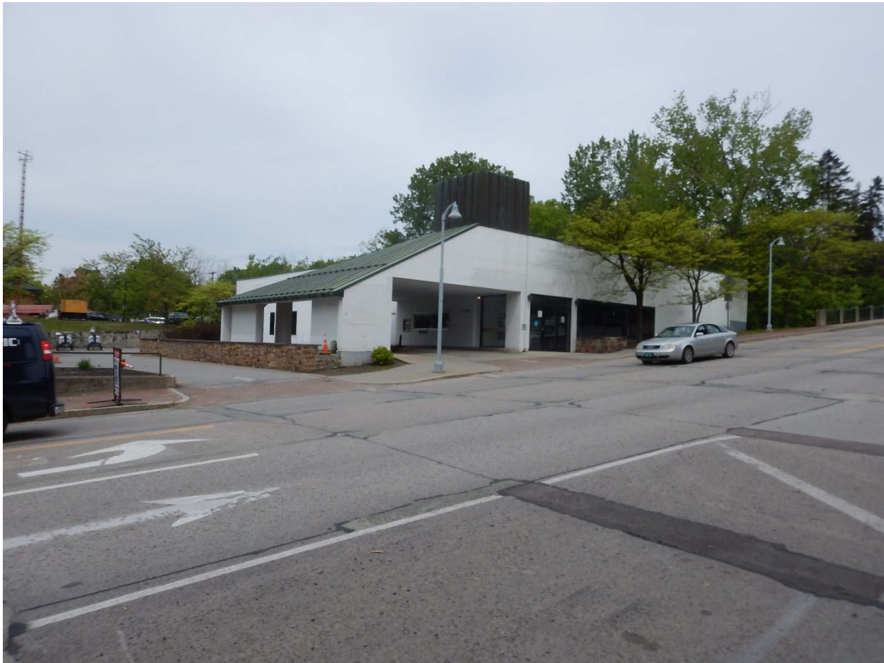
Figure 32. View looking northwest at 70 Main Street, 2017.
