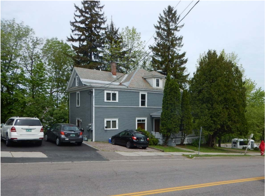
Figure 52. Looking west at 460 Colchester Avenue, 2017.
