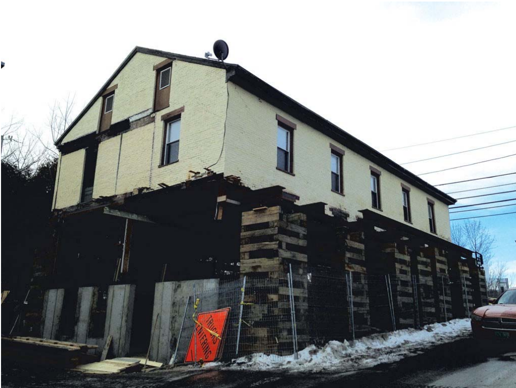
Figure 42. Lifting the second floor of 495-97 Colchester Avenue, c. 2015. View looking southwest.
