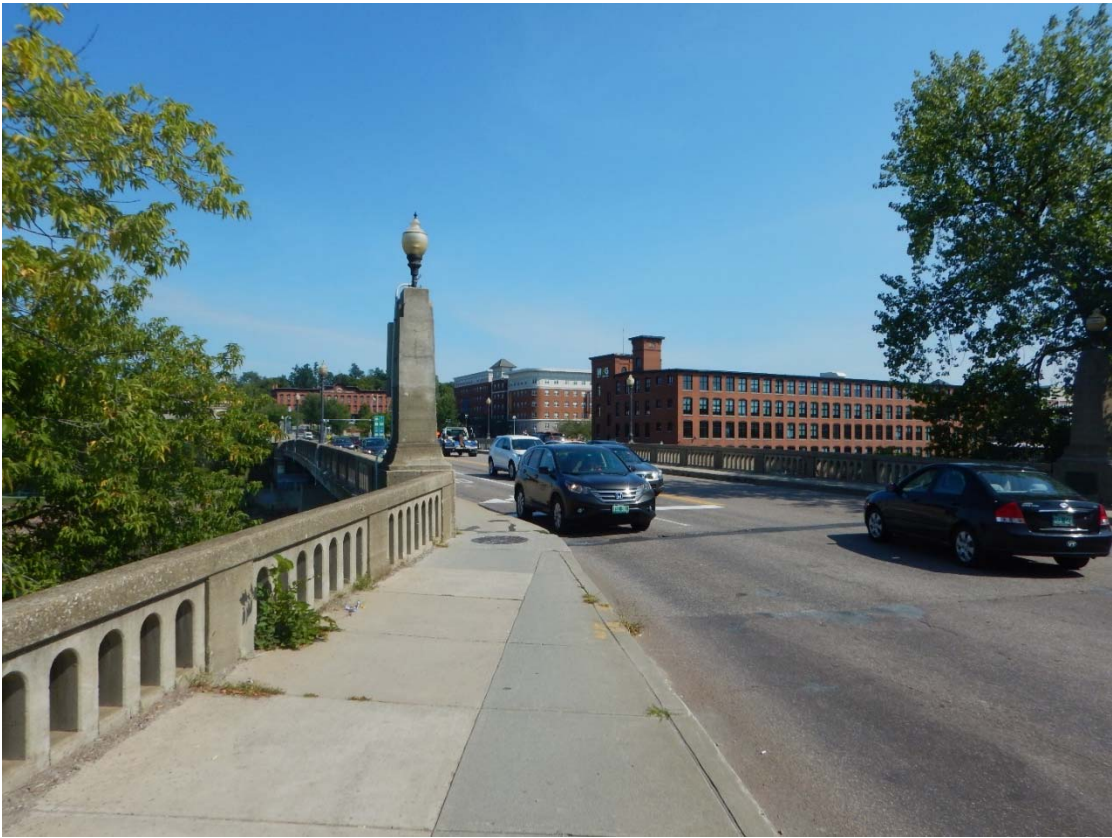
Figure 16. Winooski Bridge, detail looking north showing railing and lamp standard, 2016.
