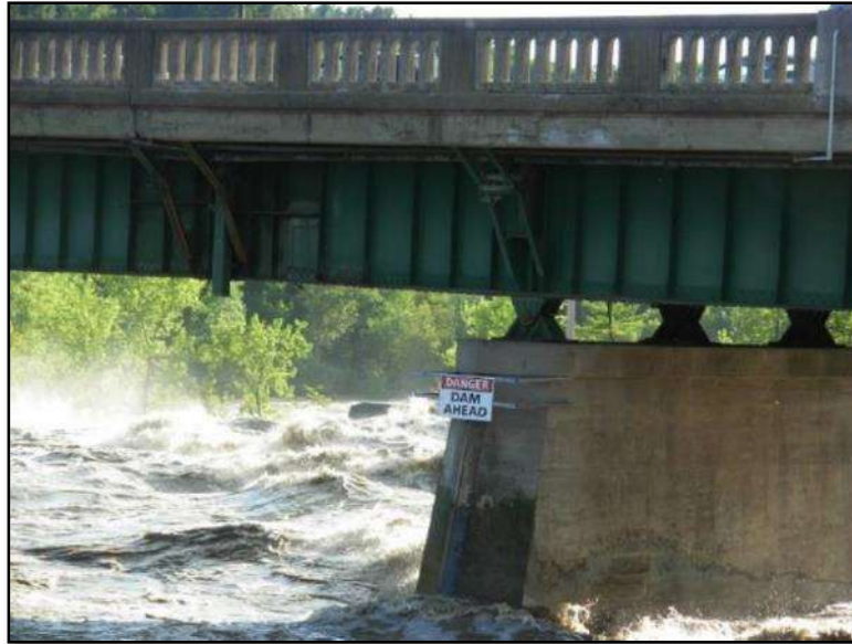
Figure 4 - Hurricane Irene (August 2011) Below the Existing Bridge
