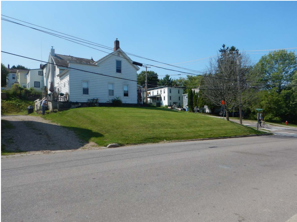
Figure 49. Looking southwest at 475 Colchester Avenue, 2016.
