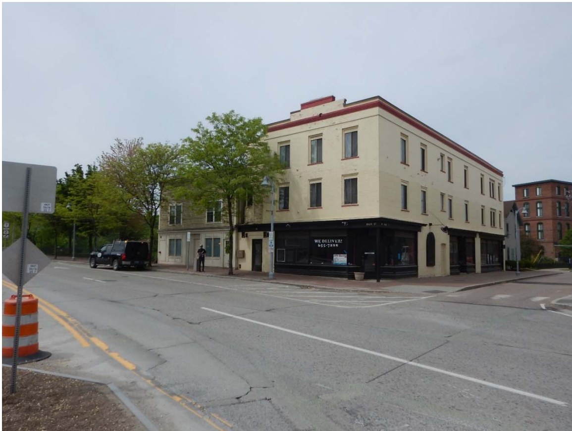
Figure 20. View looking west-southwest at 22 Main Street, 2016.
