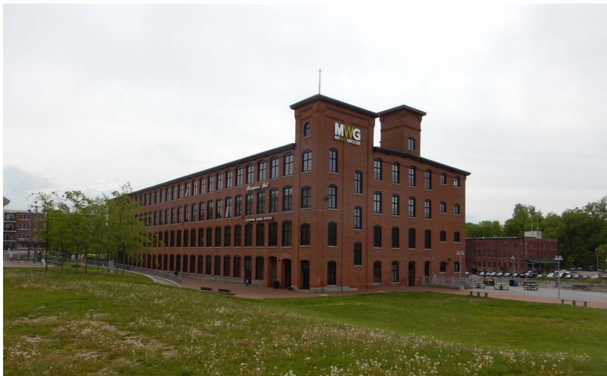
Figure 40. View looking southeast at the Champlain Mill, 2017.
