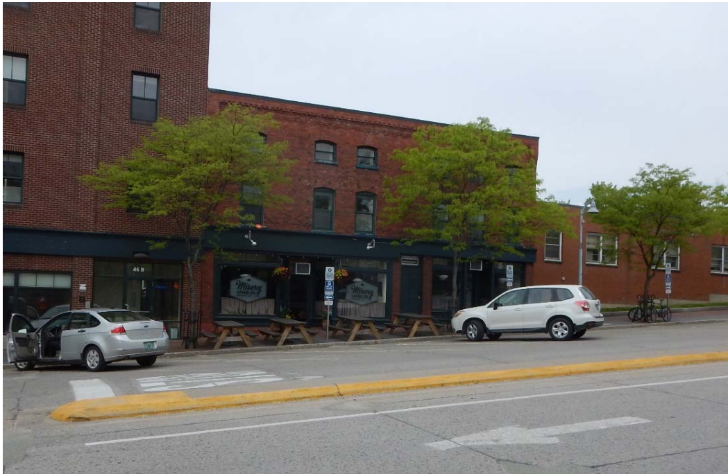
Figure 30. View looking northwest at 46 Main Street, 2017.
