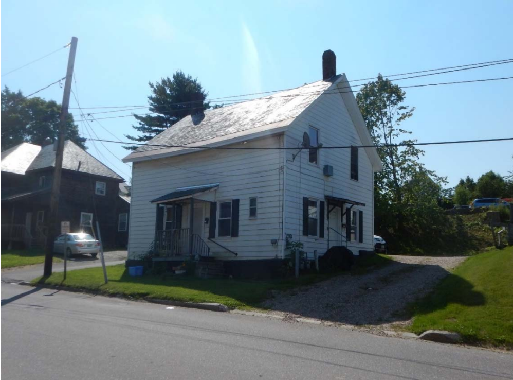
Figure 47. 11 Barrett Street, looking south-southeast, 2016.
