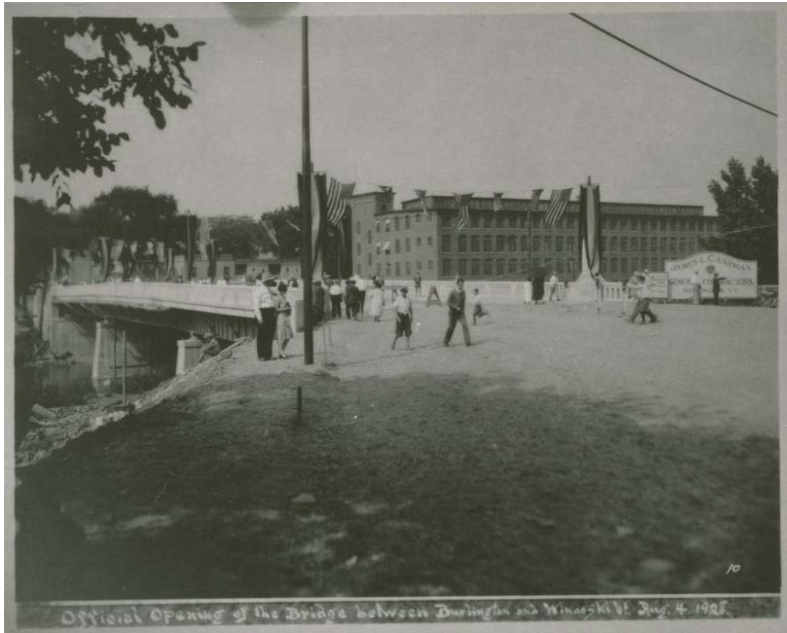
Figure 14. 4 August 1928 opening day of the bridge.
