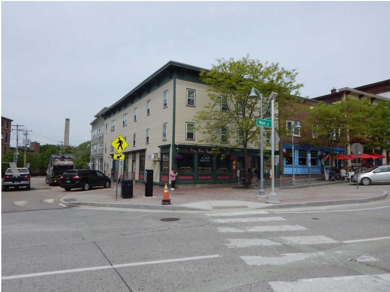
Figure 22. View looking northwest at 24 Main Street, 2017.
