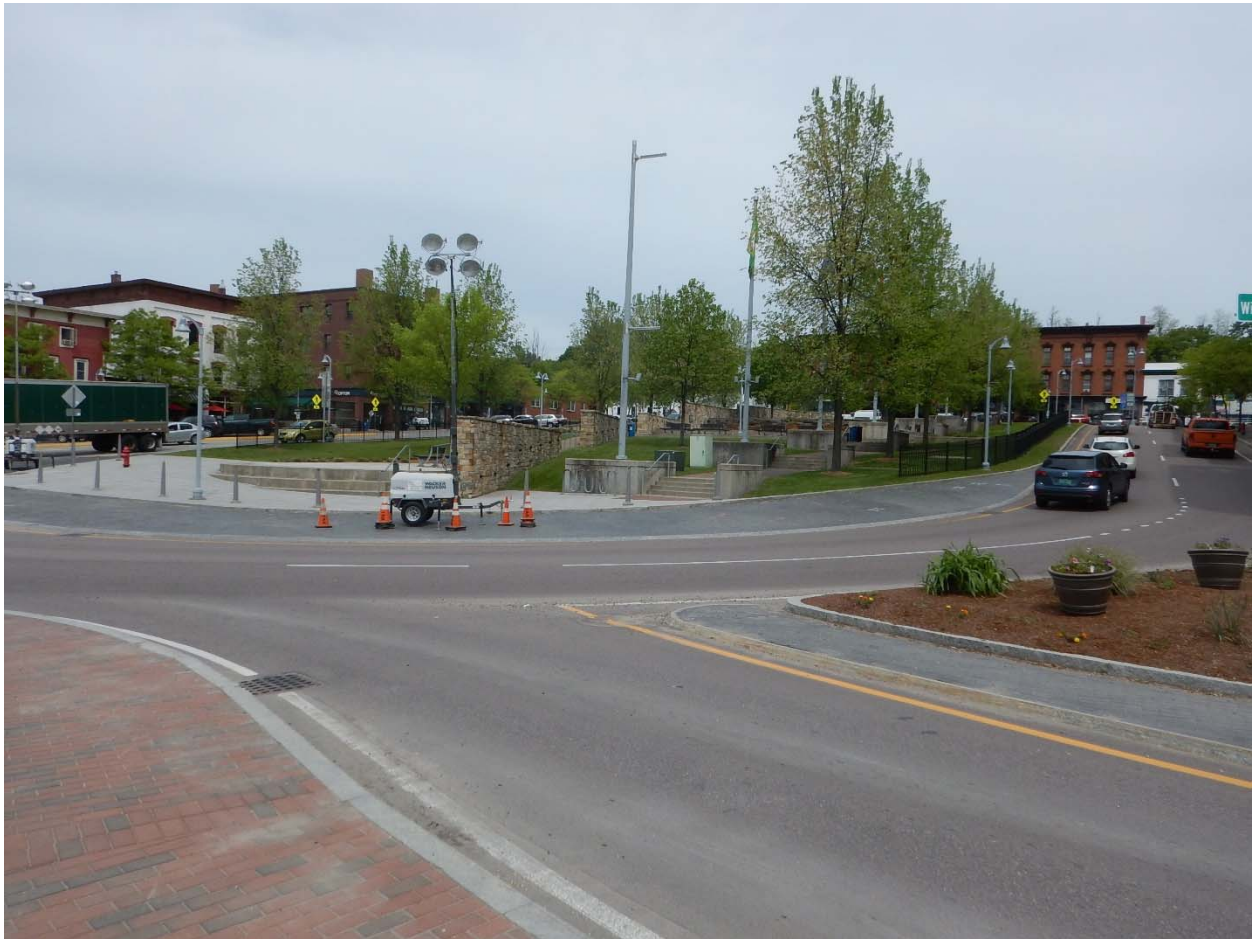
Figure 39. View looking north-northwest toward Rotary Park, 2017.
