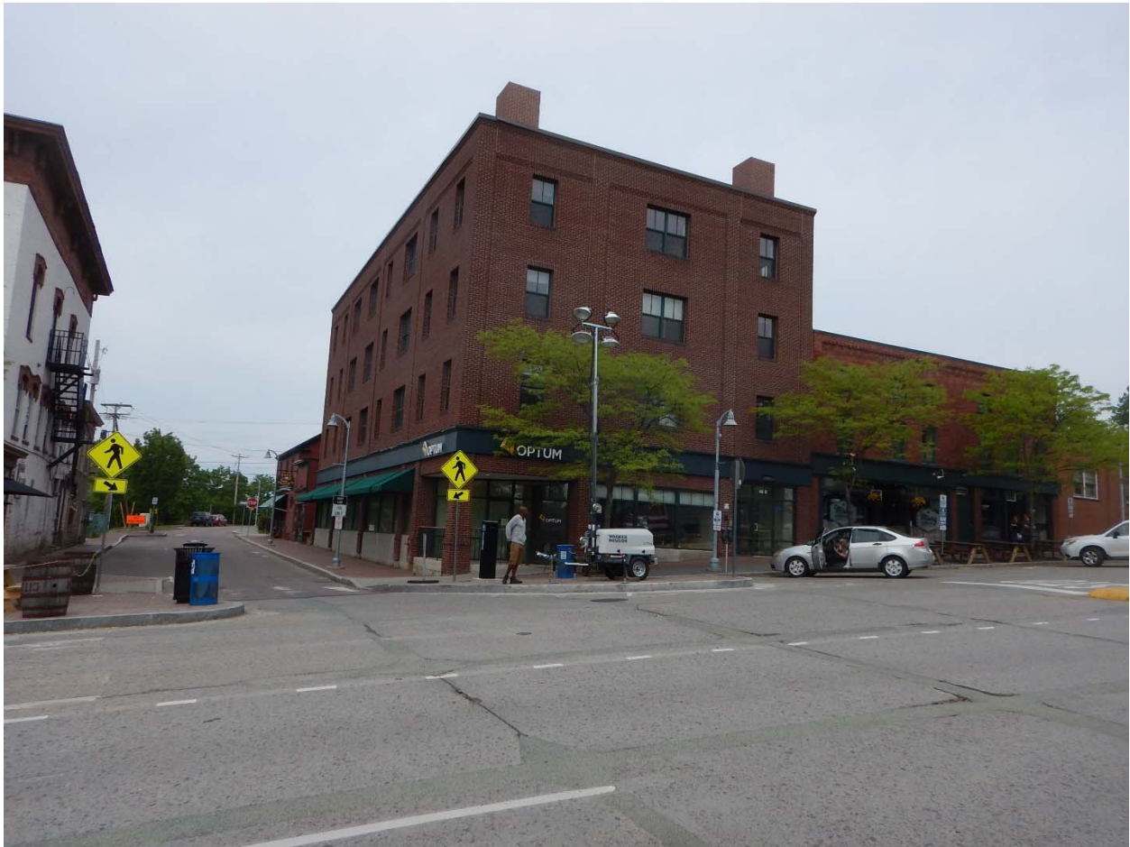
Figure 28. 40 Main Street, looking west-northwest, 2017.
