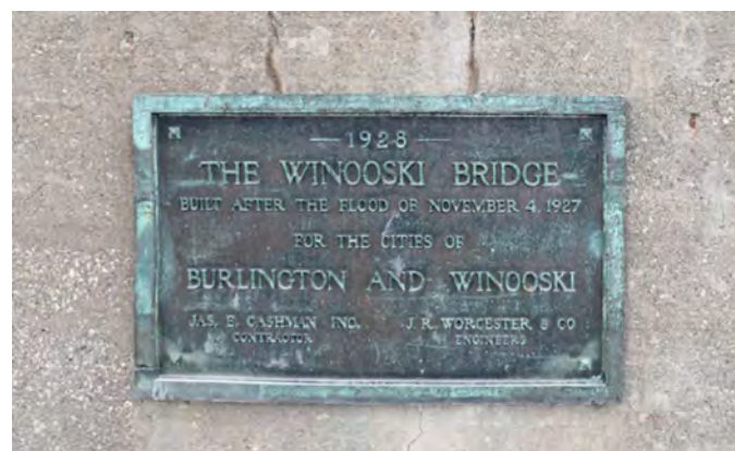
Fig. 12 – 1928 Plaque on the Parapet of the Existing Bridge
