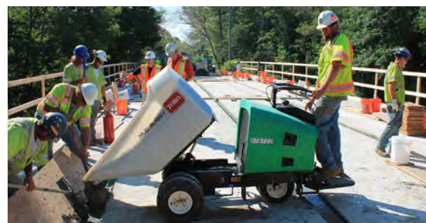
Fig. 24 - Utilizing UHPC Will Reduce The Full Closure Time for Motor Vehicles
