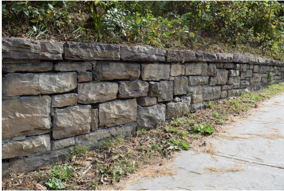
Figure 21: The stone retaining wall at Greenmount Cemetery on Colchester Avenue. To be included with the Stipulations in the RFP.
